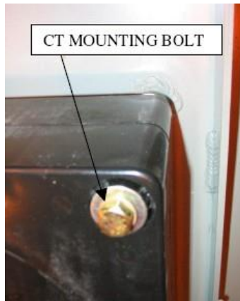
Figure 80. CT Mounting Bolt
