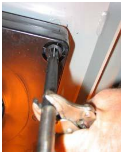
Figure 82. Reaming the Mounting Hole
