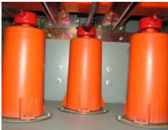
Figure 22. One Type of Metalclad Surge Suppressor
