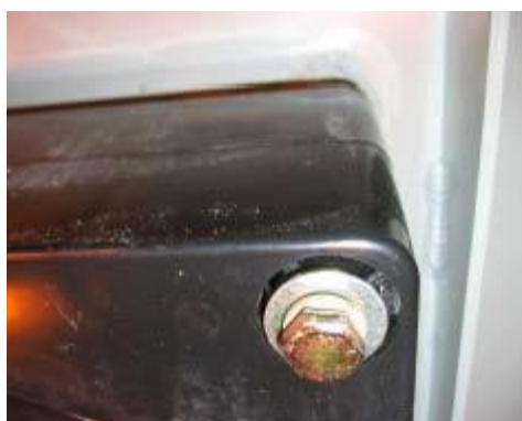
Figure 83. Newly Installed Tube and Bolt
