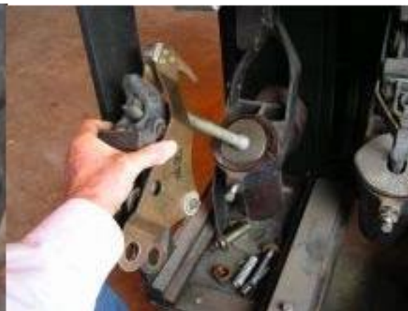
Figure 32. Lifting the Contact Assembly and Booster Piston
