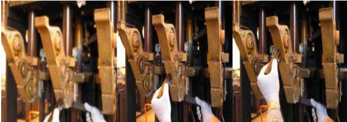
Figure 46. Testing Micro-Ohms From Stationary Primary Contacts to Arc Runners
