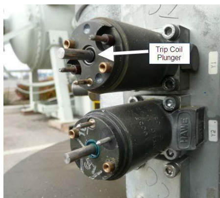
Figure 53. Trip Coil With Cover Removed
