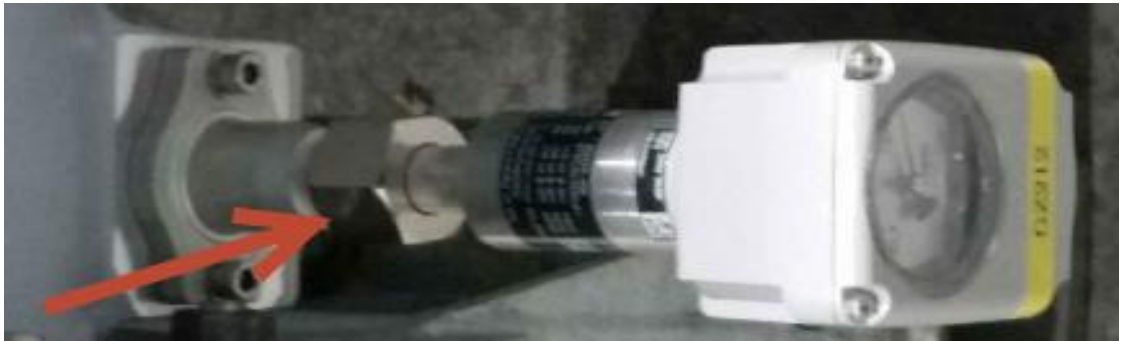
Figure 8. Trafag Density Monitor with Malmquist Fitting
