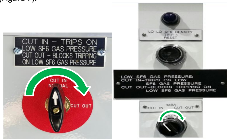
Figure 7. FCO, Lock Out Light and Reset Button
